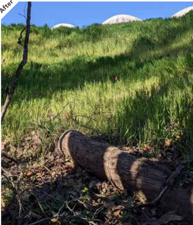
Photo point 3: Looking north, the streambank has been sloped to a 2:1. Cottonwood trees are marked with pink flags.
