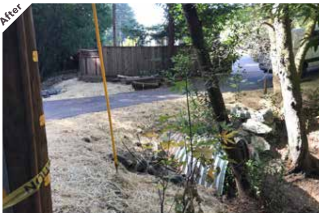
Photo point 3A: Looking downstream at the repaired crossing.
