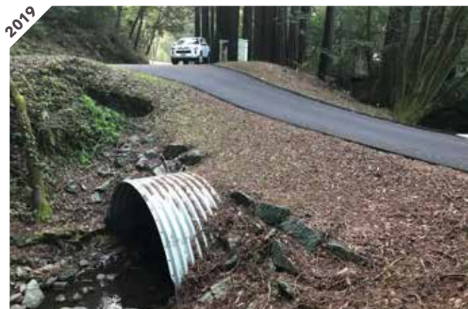
Photo point 3B: There is no erosion present at the culvert inlet. Banks are stable.
