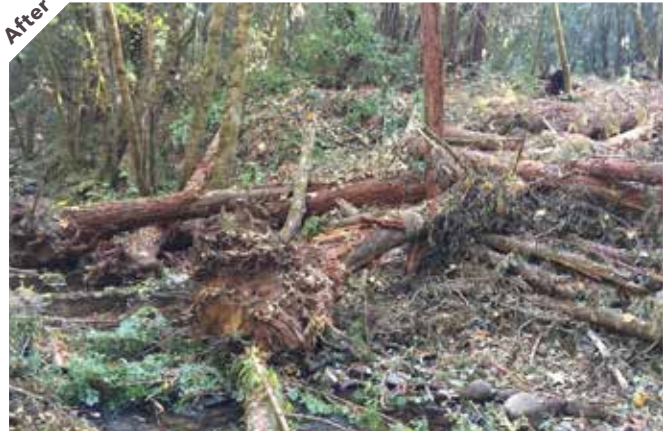
Photo point 25 - Type 2 structure. Looking upstream. Structure ultimately built slightly upstream of where pre-photo taken. Rocky bank visible in lower right of the photo. Rootwads visible.
