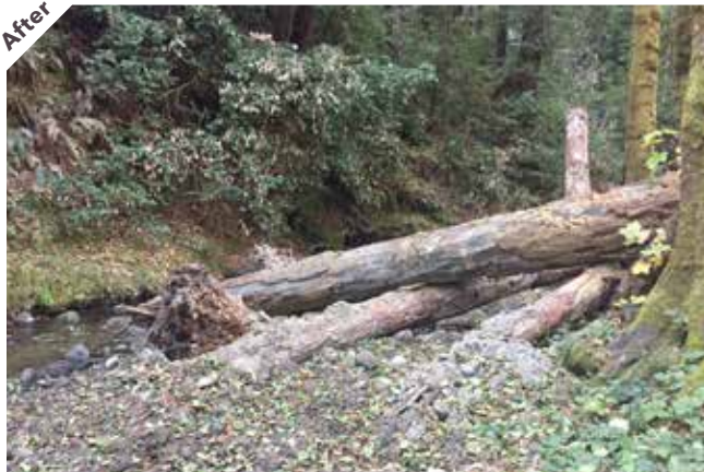
Photo point 20: Looking downstream at Type 1 structure. Rootwads visible.
