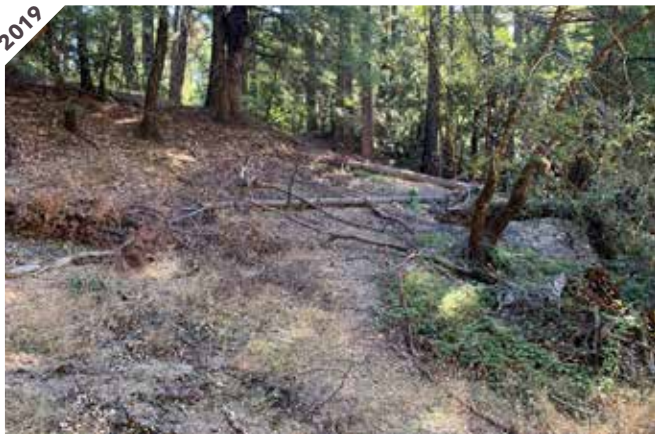
Photo point 9: Looking east uphill at former road junction. Decommission is effectively reducing runoff.
