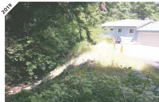
Photo point 2: Looking south at the top of the bank failure. The site is stabilized and revegetated.
