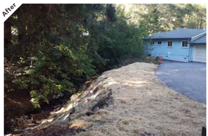
Photo point 2: Looking at the top of the bank failure. The site has been seeded and mulched.
