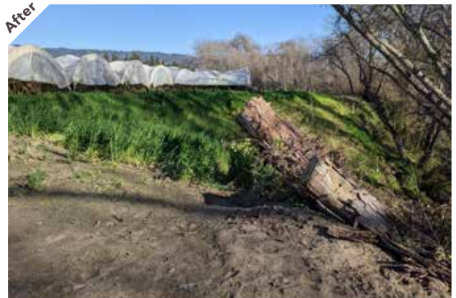
Photo point 2: Looking east, the bank has been sloped and well-seeded with common barley.
