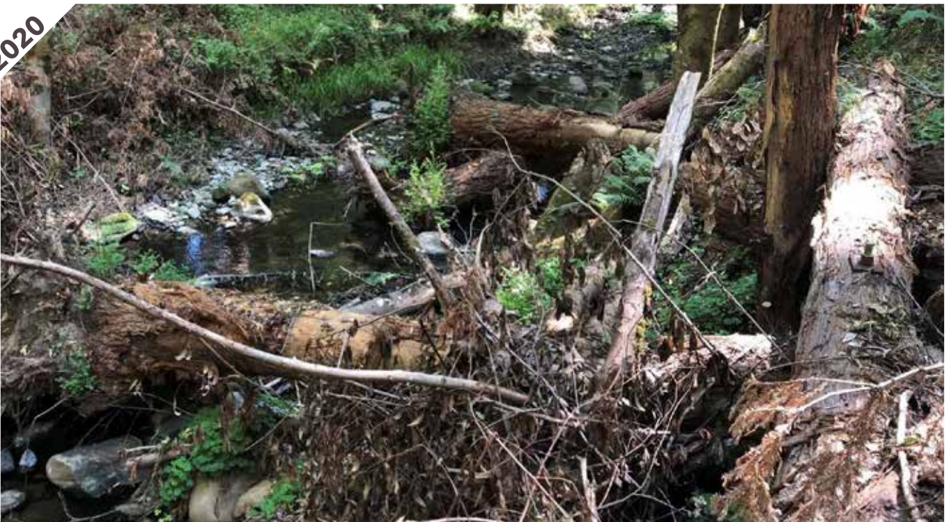
Photo point 25: Type 2. Looking upstream. Structure ultimately built slightly upstream of where pre-photo taken. Rocky bank visible in lower right of the photo. Rootwads visible, and sprouting in creek. No significant pooling present or changes in morphology.
