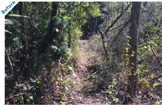
Photo point 5: Standing on and looking south across the failing embankment. The low spot/scour area is visible just before the stake on the downstream side of the embankment.
