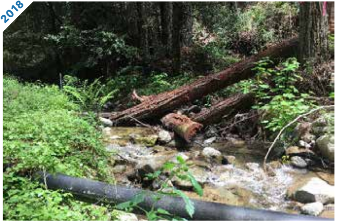
Photo point 5: Large wood was placed and a notch carved into the side channel to initiate floodplain re-activation.
