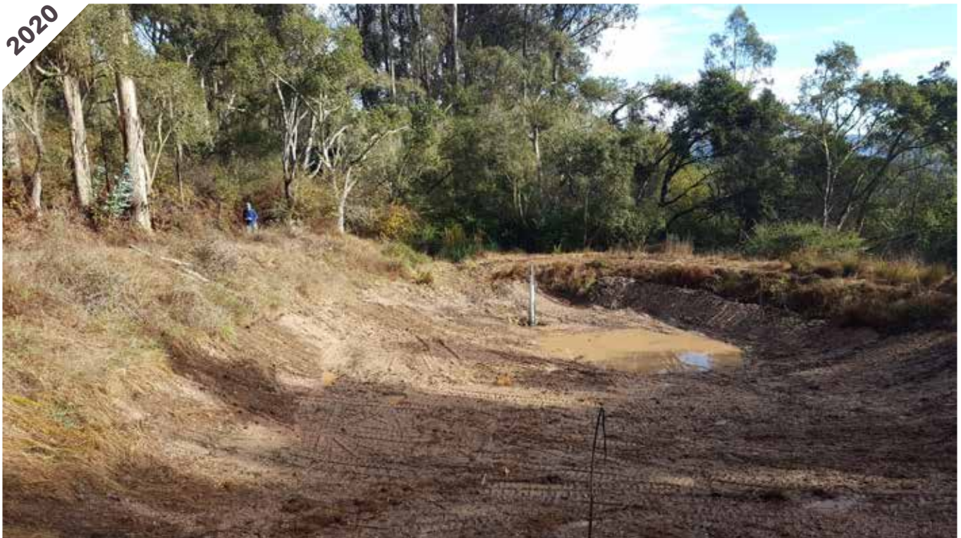
Photo point 3-2: Juncus and other wetland plants were undisturbed during pond lining. All topsoil was replaced.
