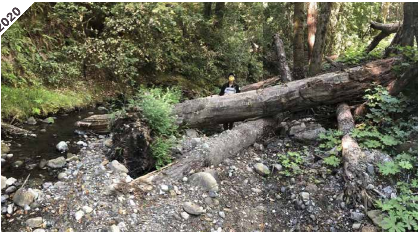
Photo point 20: Type 1. Looking downstream at Type 1 structure. Rootwads visible and are sprouting. No significant wrack up visible due to low flow events in 19-20 wet
