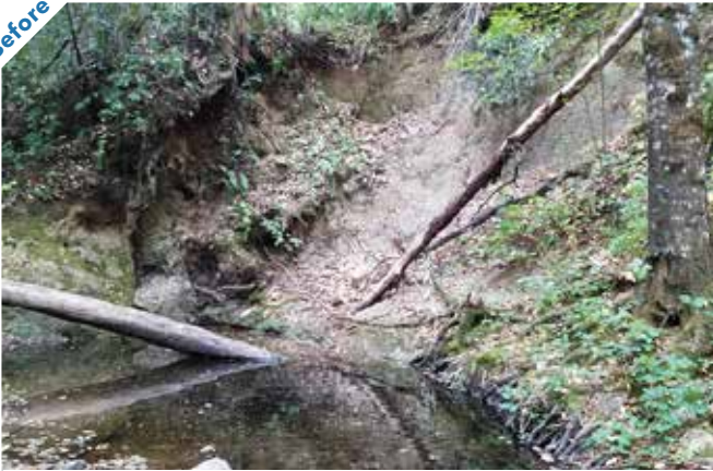
Photo point 23: Looking upstream at future location of structure. Historic landslide visible as well as bedrock.
