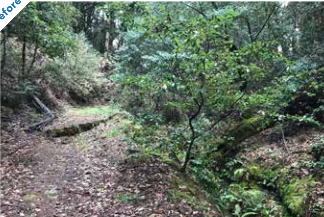
Photo point 5: Looking up the old access road that was decommissioned. Notice the road failure from concentrated runoff and a fallen tree.
