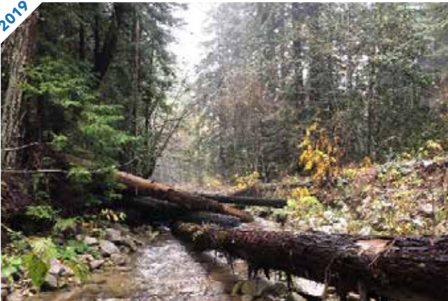
Photo point 5D: Large wood, placed just upstream of the confluence of San Vicente and Mill Creeks, is creating deposition.
