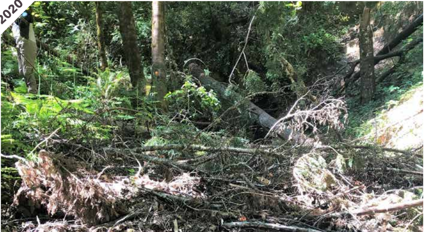
Photo point 23: Type 3. Looking downstream at Type 3 structure. Historic landslide visible still slightly visible in background, bedrock hidden by branches. Pooling on downstream end of structure. Significant wrack up occurring of small branches at upstream end. Bank vegetation grown in significantly.
