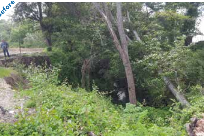
Photo point 2: Looking east, the eroded, scalloped edge of the streambank can be seen on the left side of the photo.
