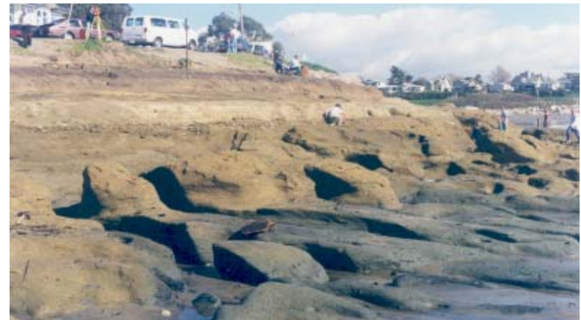
Danger to road & utilities,
