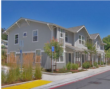
Parkhurst Terrace, affordable apartments
