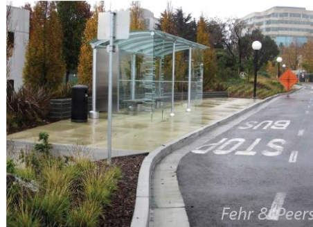
Bus shelter with passenger amenities.
