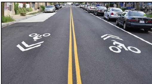
Sharrow road markings. Photo credit: locallygrownorthfield.org
