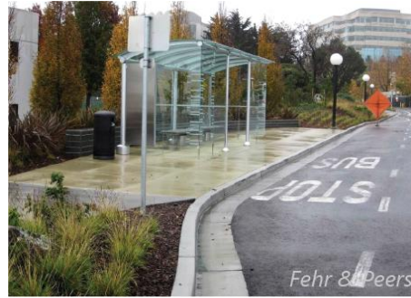
Bus shelter with passenger amenities. Photo credit: Fehr & Peers, 2014
