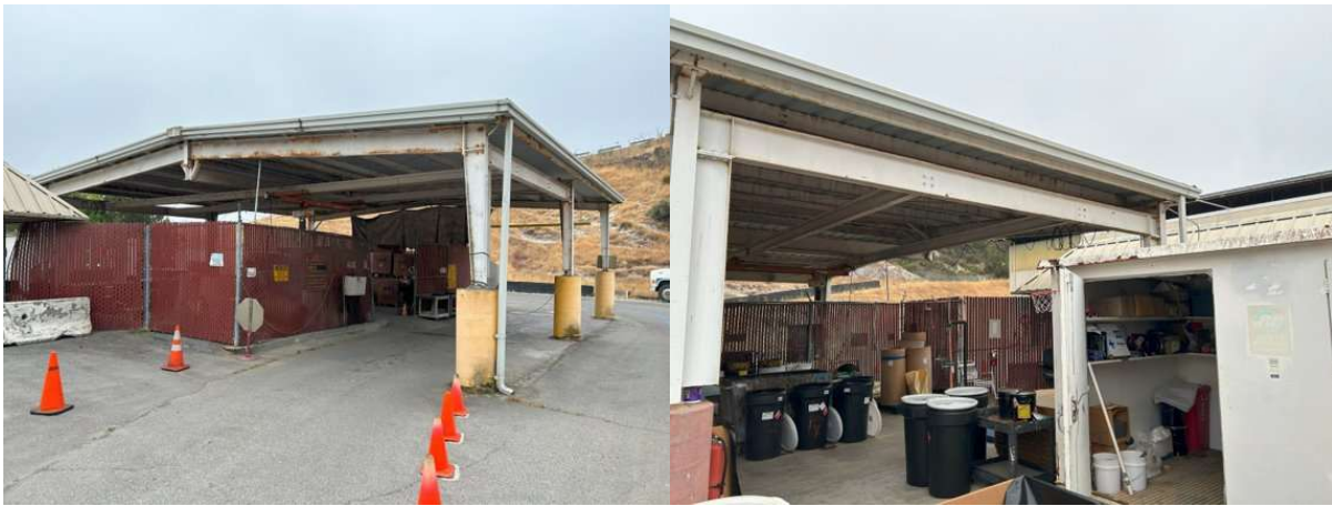
The existing Ben Lomond HHW collection area prior to construction of the HD44-funded facility improvements.
