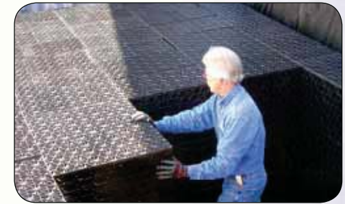
Underground systems can be customized to fit various shapes and sizes using these modular RainBoxes.
