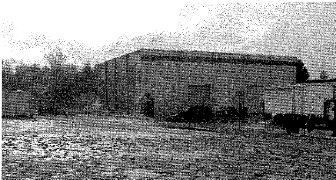
Figure 1 - Photo shows runoff from the property flowing west across the rear property line
