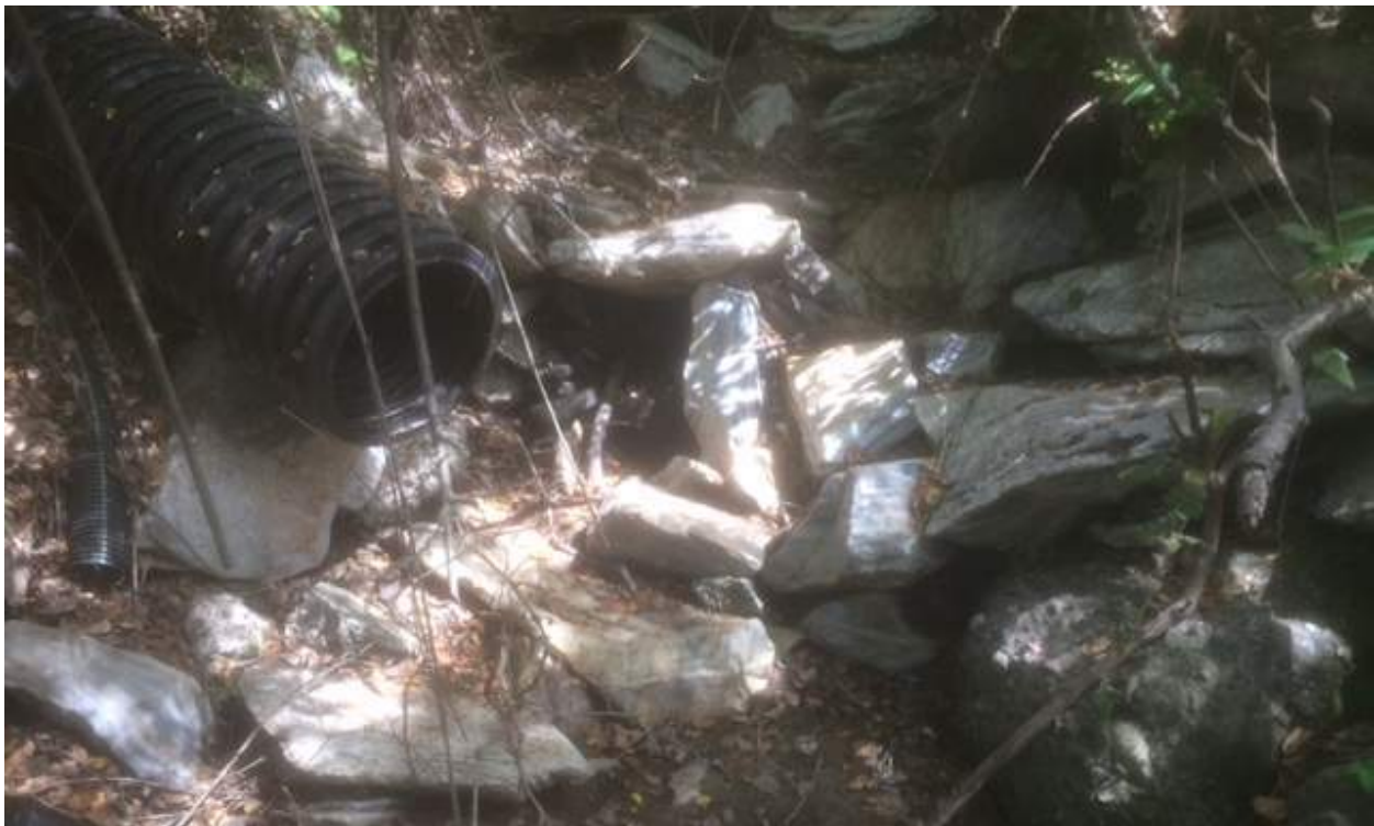
Figure 5- 15" CPP Culvert Discharge Point
