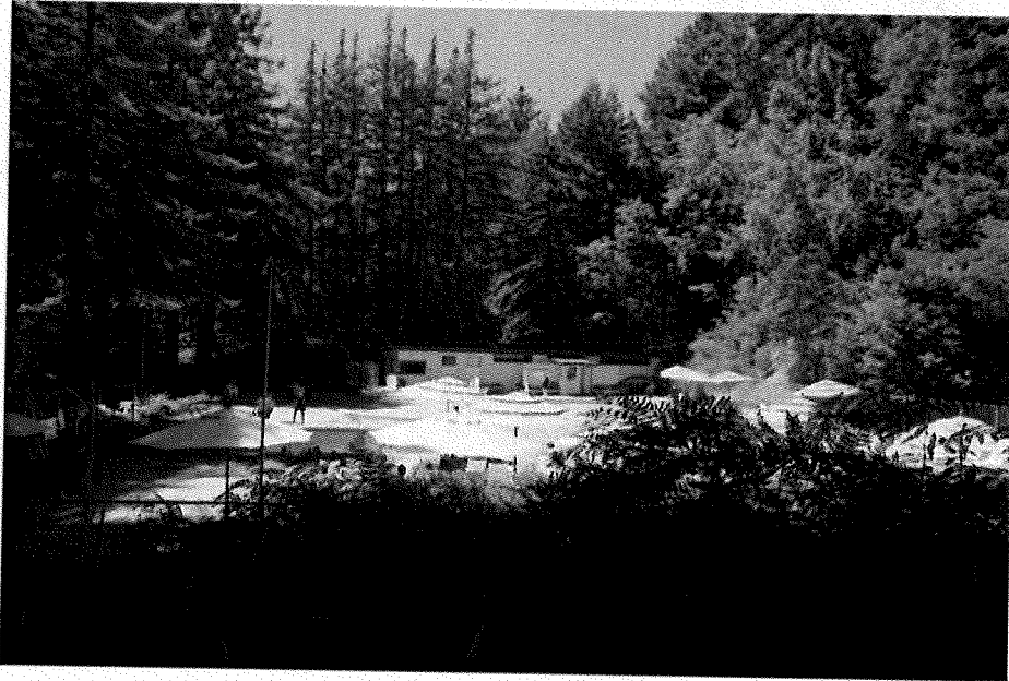
Figure 22: Pool and pool house, 2016.
