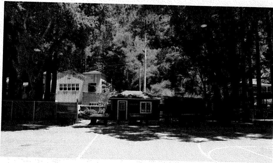
Figure 11: Maintenance Office front façade, 2016.
