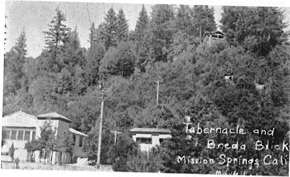
Figure 10: View of the Tabernacle from the approximate location of the present day Maintenance Office. Source: Mission Springs, 1944.
