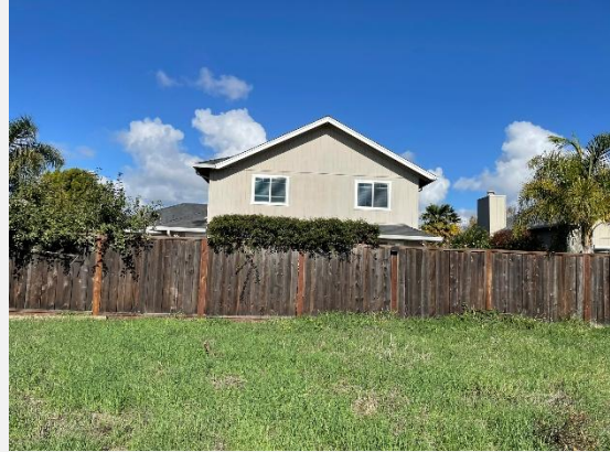
Photograph 14. Northern adjoining residential housing.
