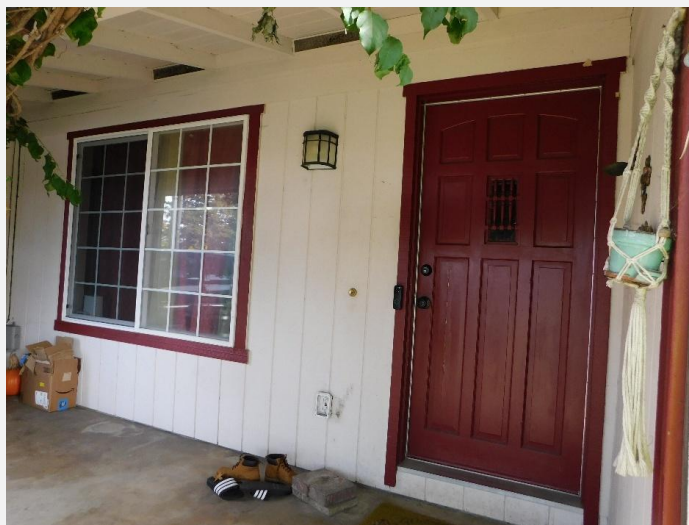
Photo 2. Detail photograph of the west elevation's front porch, camera facing east.
