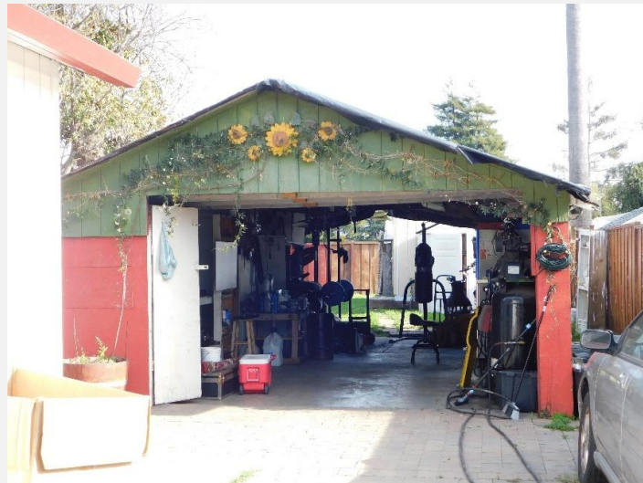
Photo 4. Detached garage, camera facing east.
