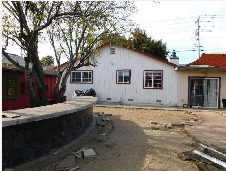
Exhibit 9. Rear (east) elevation showing replacement windows and door, camera facing west.
