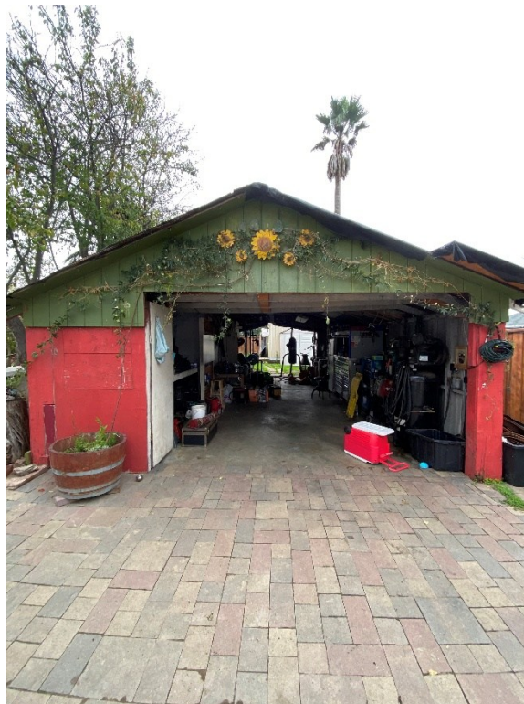
Exhibit 12: Overview of garage structure at 2030 17 th Avenue. View E 100°.
