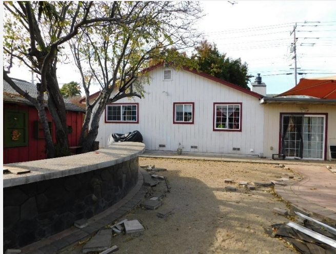
Photo 3. Rear (east) elevation showing replacement windows and door, camera facing west.
