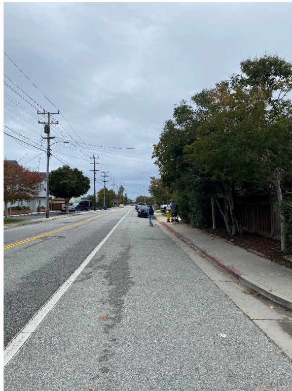
Exhibit 16: Overview of 17 th Ave Right-of-way from northern boundary of APE. View S 198°.
