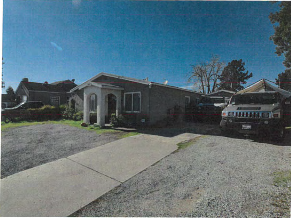
Front façade, viewed facing southwest.
