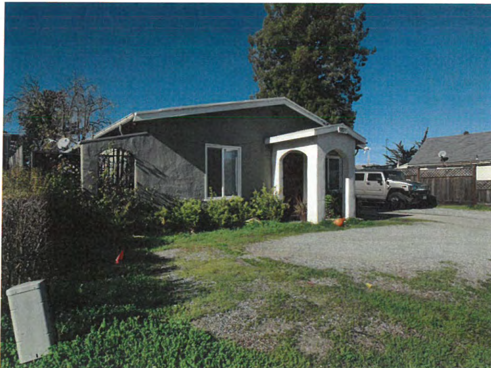
Front facade, viewed facing northwest.
