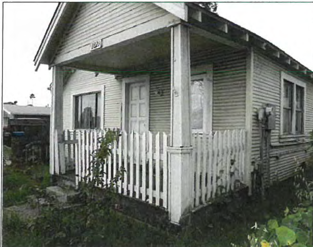
Photo 5: Residential structure along 41 st Street.
